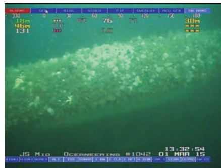
West horizontal bracket, with dense blue mussel, hydroids, frilled anemone and sea stars
