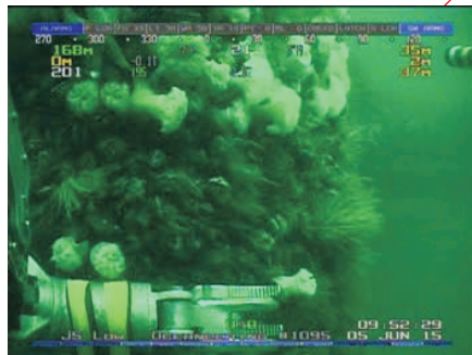
Dense mussel with hydroids and frilled anemone at MG 10, on the lower part of Leg 4
