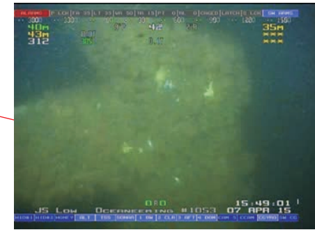
Mussel with hydroids on top, and occasional sea stars at the top of Leg 2.
