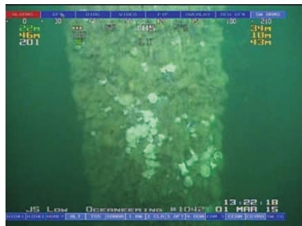
Mid-way up Leg 1. Dense mussel, covered in hydroids, frilled anemone and sea star.
