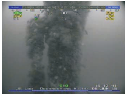
Dense mussel and hydroid on Anode 7 on Leg 3.
