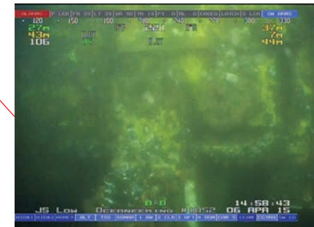
Blue mussel and hydroids on the subsea tree.
