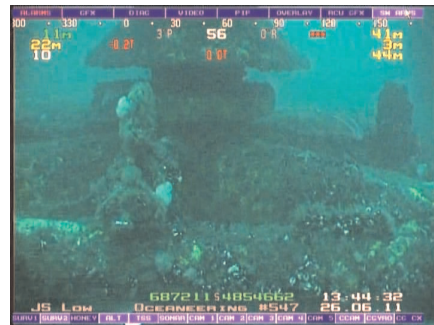
Algal growth and mussels at base of Subsea Tree
