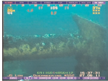
West horizontal brace with few patches of blue mussels
