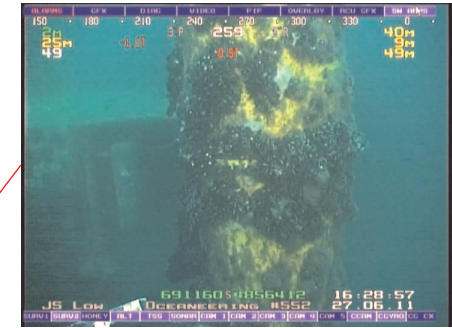
Patches of blue mussels and sea anemone on upper section of Leg 2
