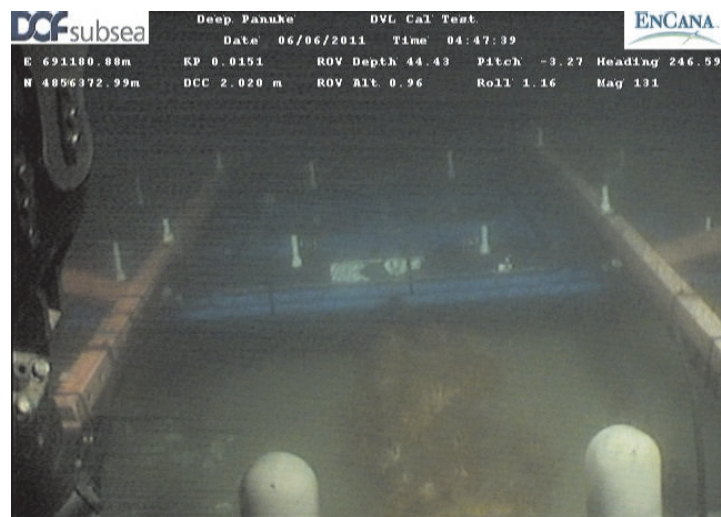
Exposed flowline to wellhead D-41 with 100% fouling of the sea cucumber Cucumaria frondosa
